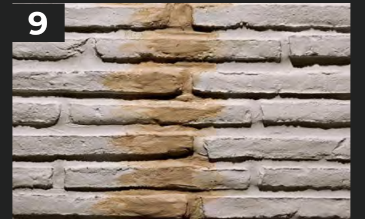
9. Spachtelmasse trocknen lassen Waiting for drying for assembly putty
