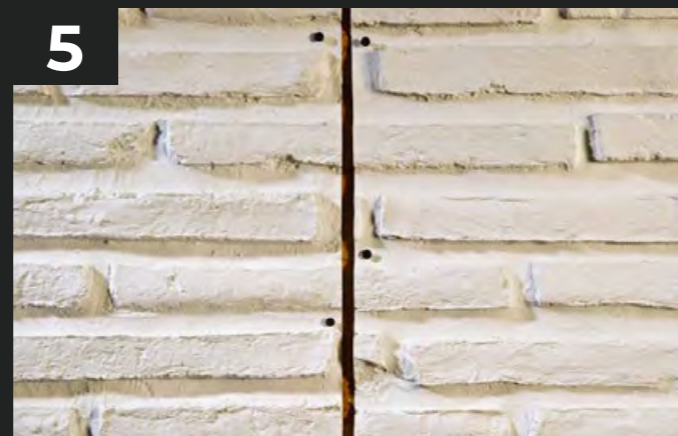
5. Abstand von ca. 1 cm zwischen den Paneelen frei lassen Leaving a space by 1 cm between two panels
